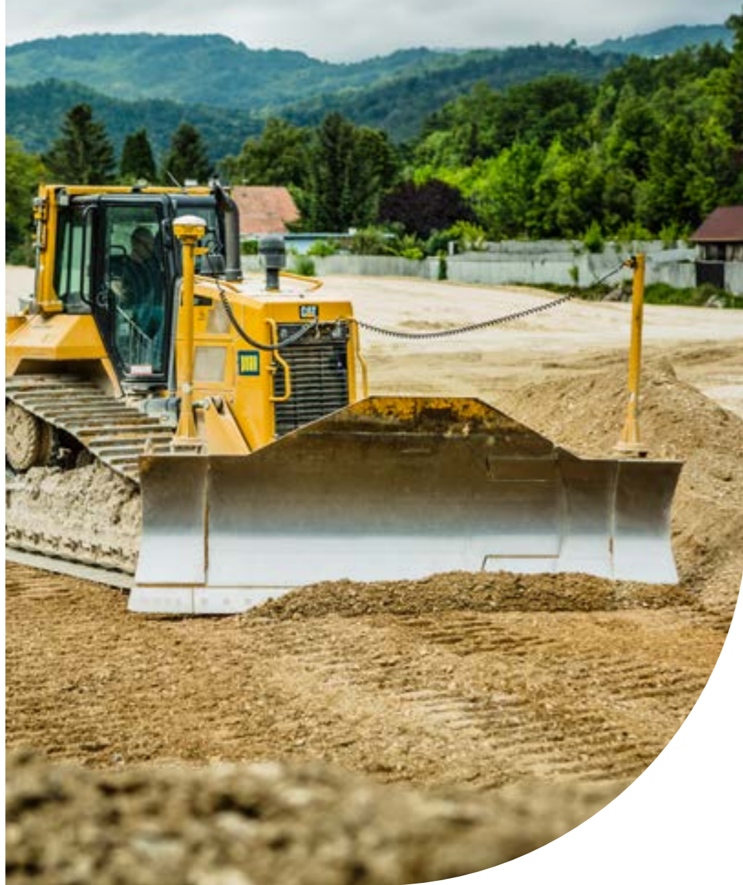
Flood retention basin Fahrafeld/Lower Austria – Austria Earthworks at the largest retention basin in Lower Austria
