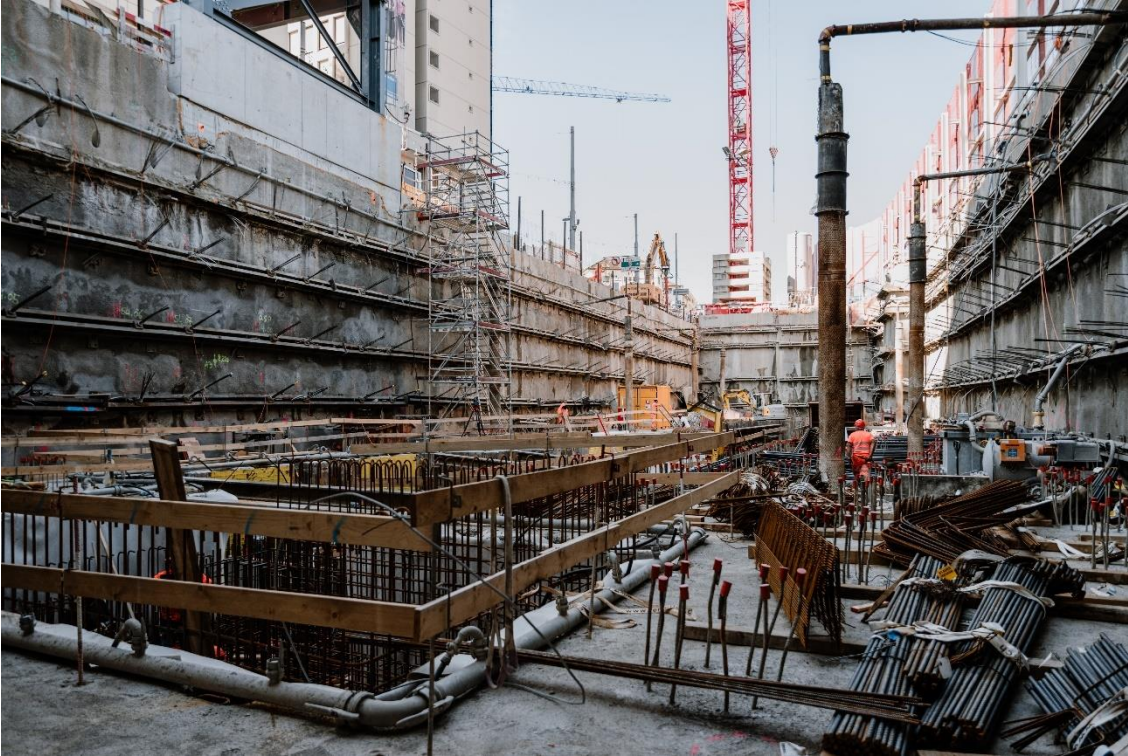
Caption: Excavation pit of the Franklinturm in Zurich-Oerlikon © PORR
