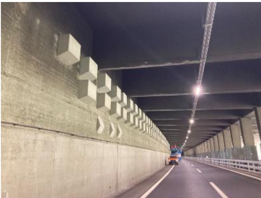
Figure 2: Anchor head renovation Ripplistahl gallery (141 units)
