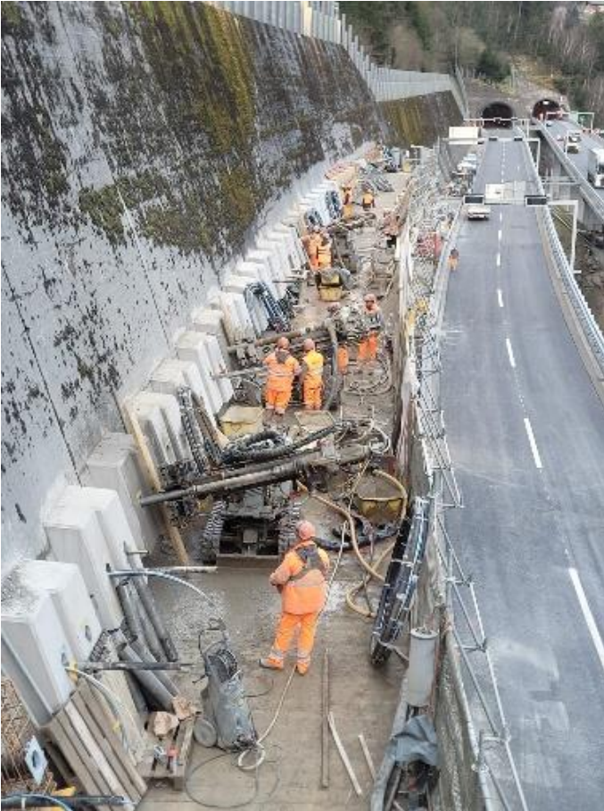
Figure 3: Höll retaining wall Anchor heads and strand anchors
