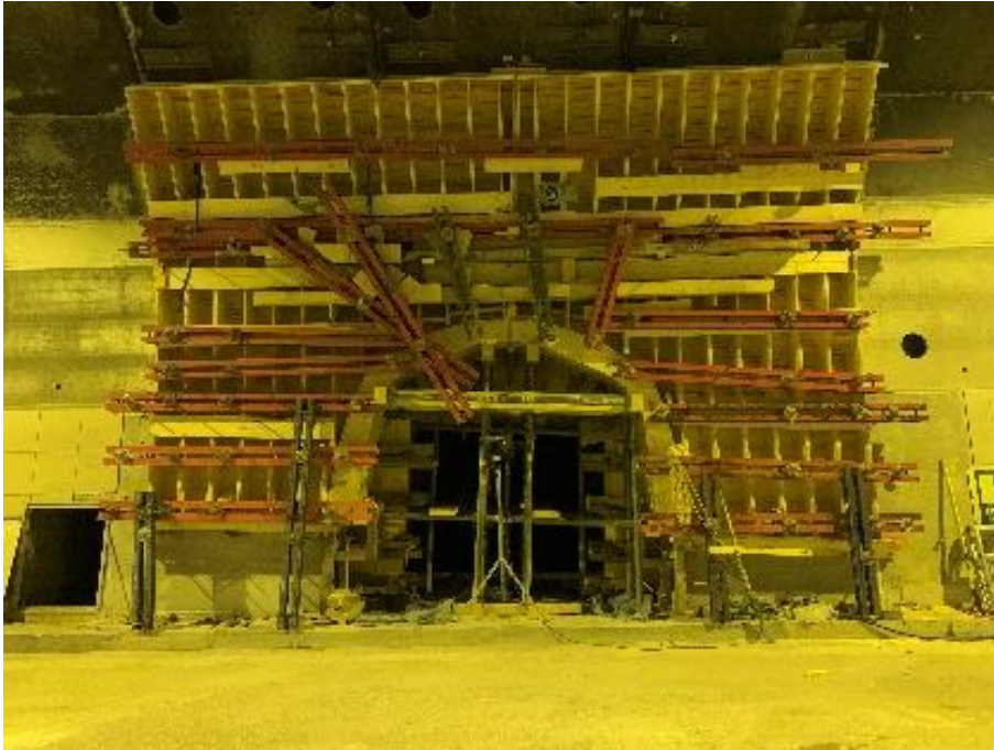
Figure 1: Cross connection Platti Tunnel parament formwork in the main tunnel FBSU
